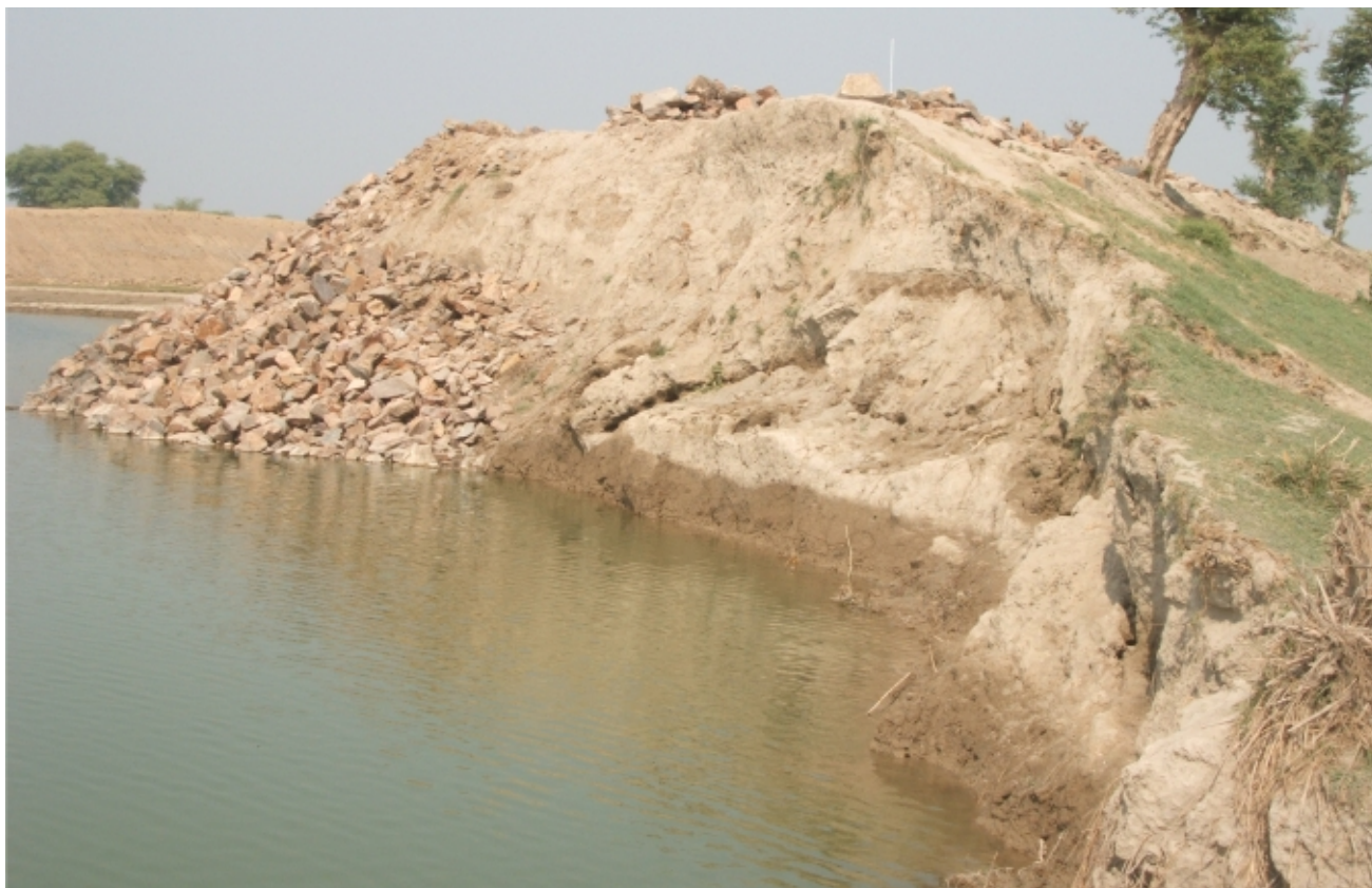
Photo showing face of un-pitched breach section at RD 39+000
