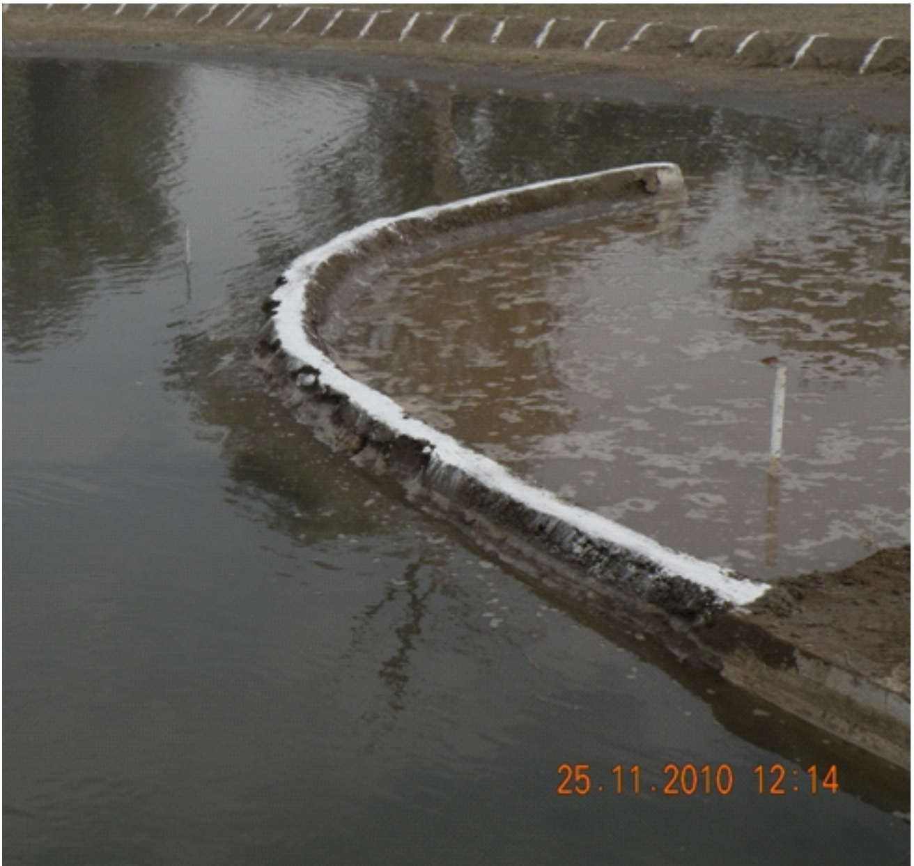
Normal Operation of Barrage at Q = 3,00,000 Cusec
